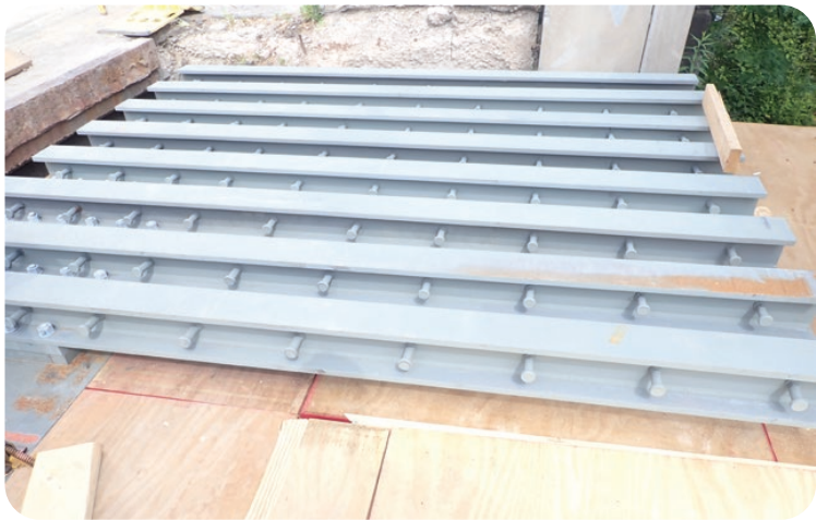
Deck beams in Span 1 to help support the north overhang at the acute corner of the West Abutment.
