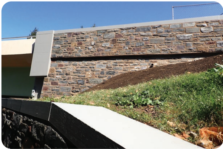
East abutment wingwall where existing stones were reused wherever possible.
