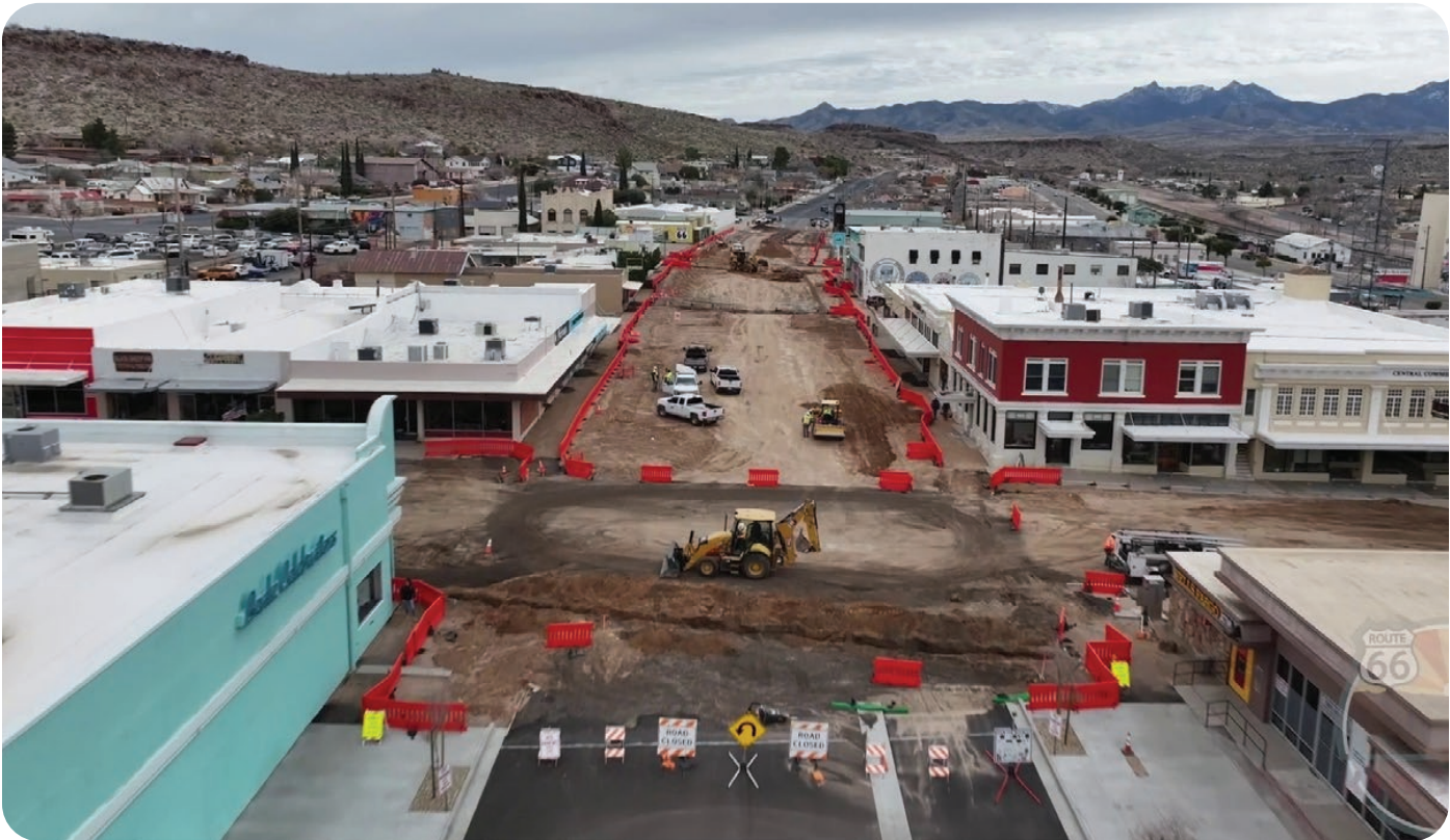
One of the main Beale Street intersections during the construction phase of the project.
