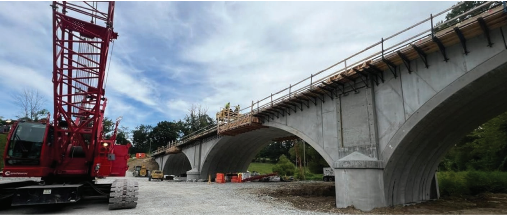
Deck construction and precast spandrel wall panels completed.
