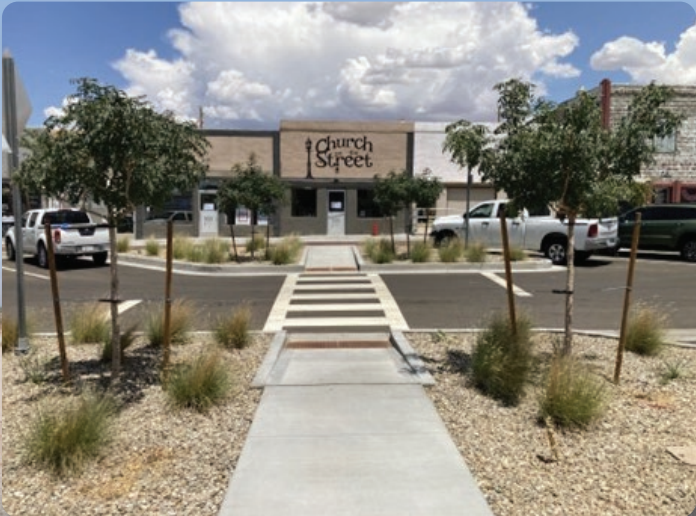
One of the high visibility crosswalks that were added as a part of this project.
