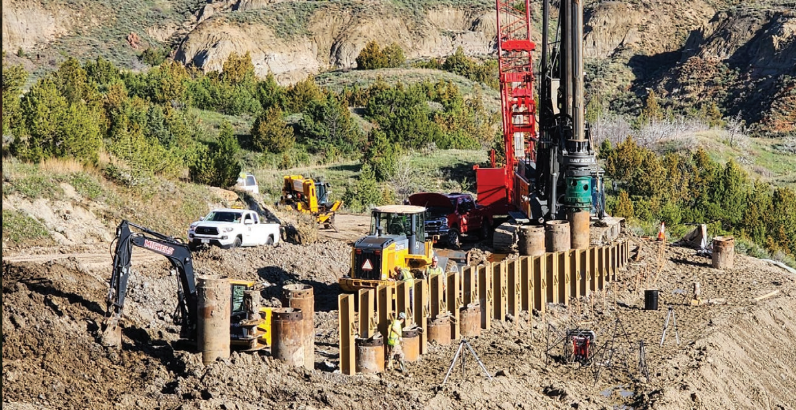
Installation of second row of drilled shafts.
