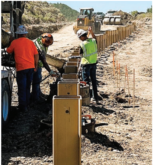
Encasement of vertical steel soldier piles in concrete.
