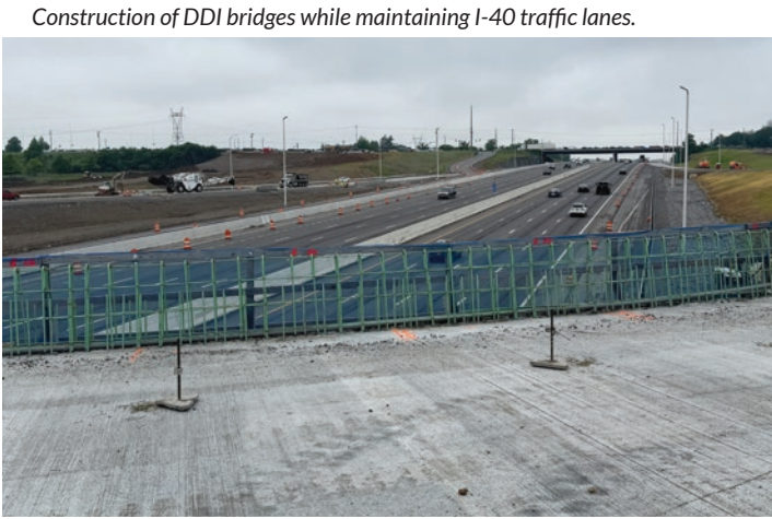
Construction of DDI bridges while maintaining I-40 traffic lanes.
