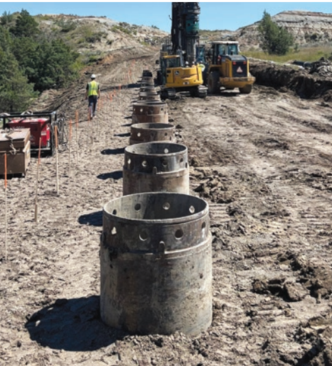
Drilled shafts prepared for concrete encasement.
