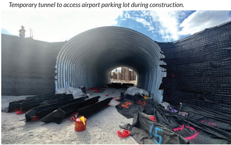
Temporary tunnel to access airport parking lot during construction.
