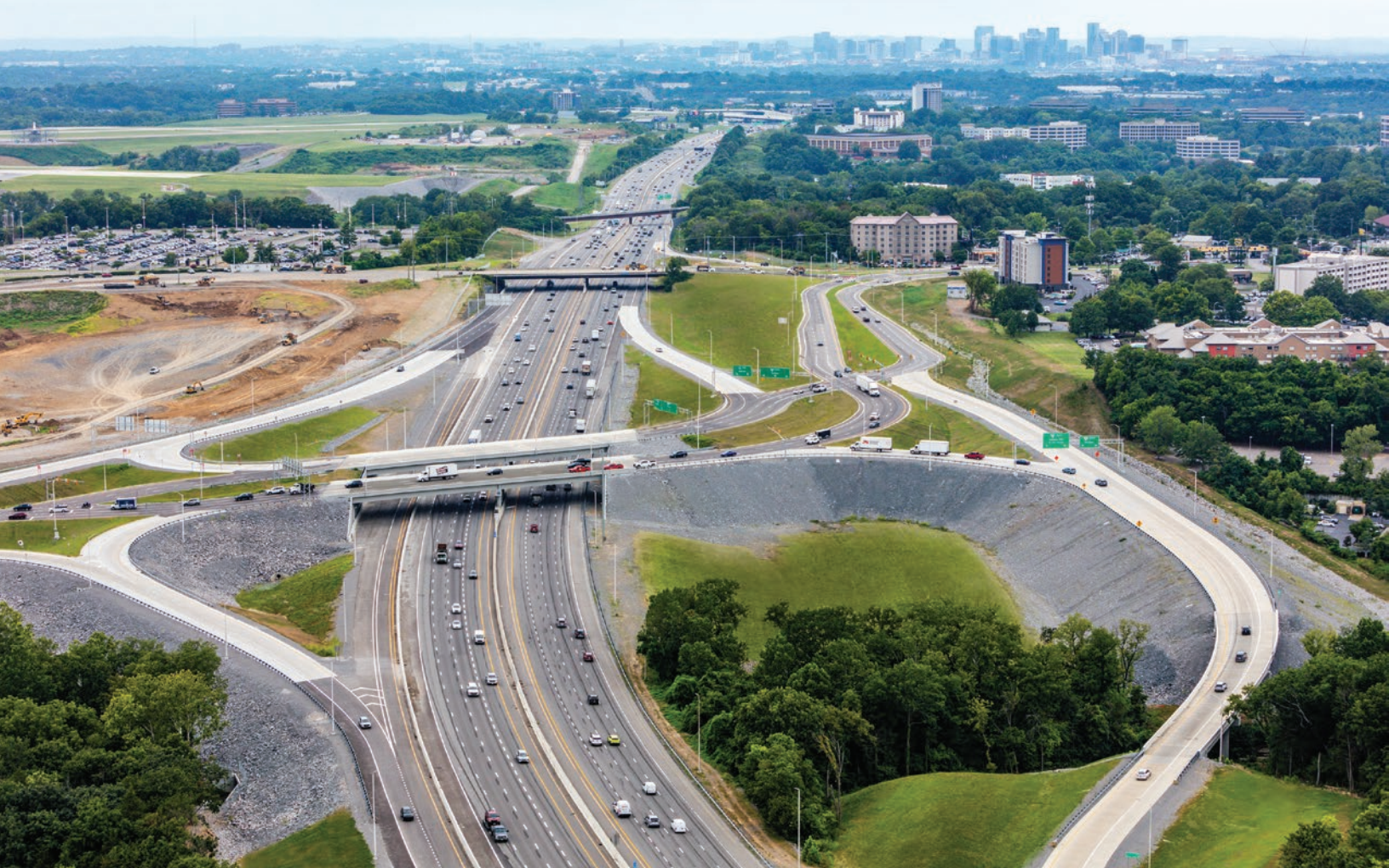
New Donelson Pike DDI greatly improves vehicular access between airport and downtown Nashville.
