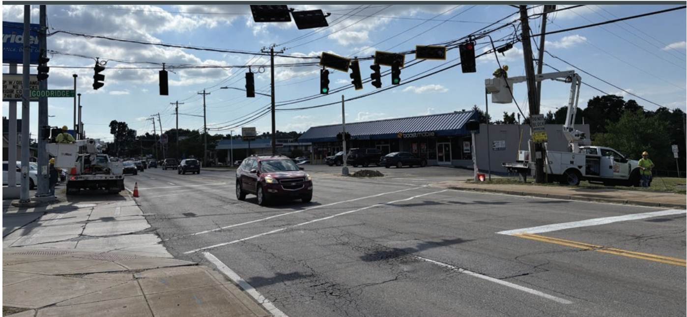
Signal head upgrades being installed at the intersection of US 25 and Goodridge Dr.
