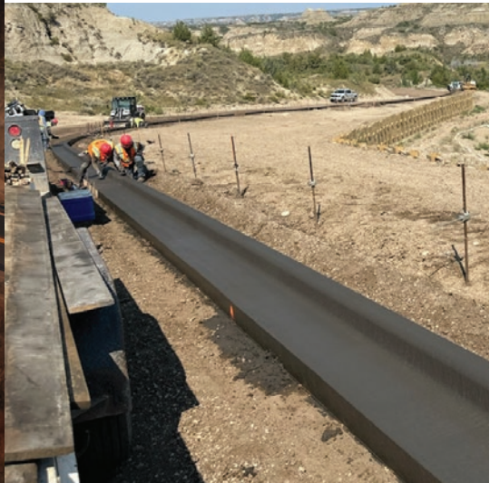
Freshly placed concrete curb along the scenic loop.
