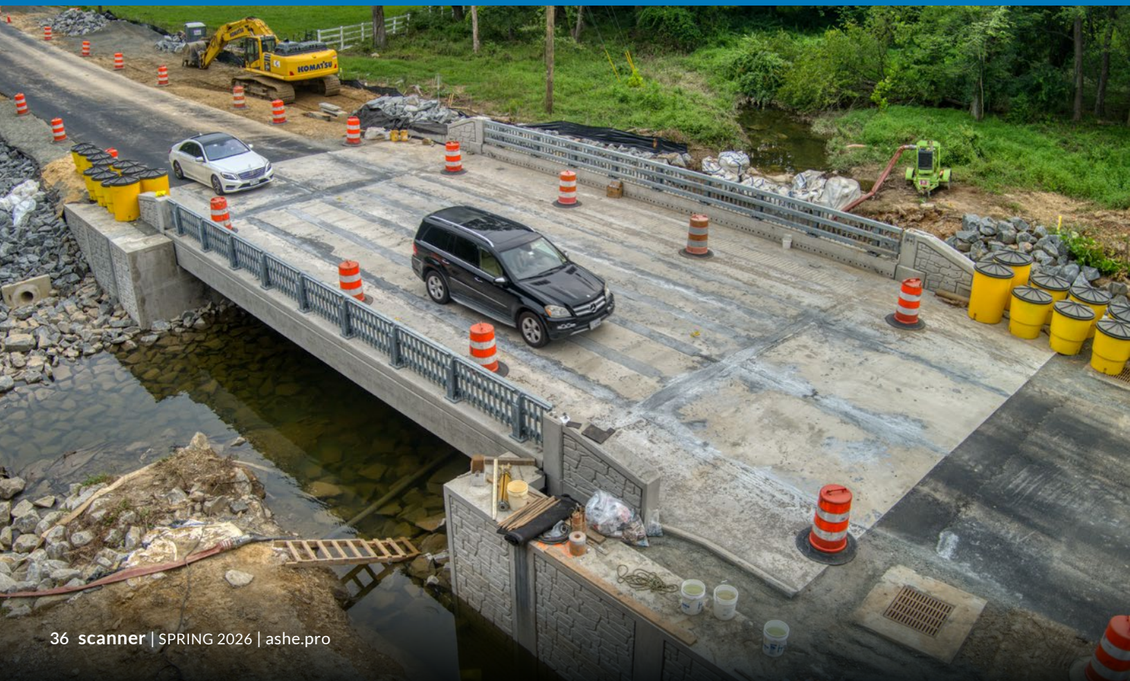
Top: Superstructure precast units being put in place Bottom: New bridge open to traffic during final construction stages
