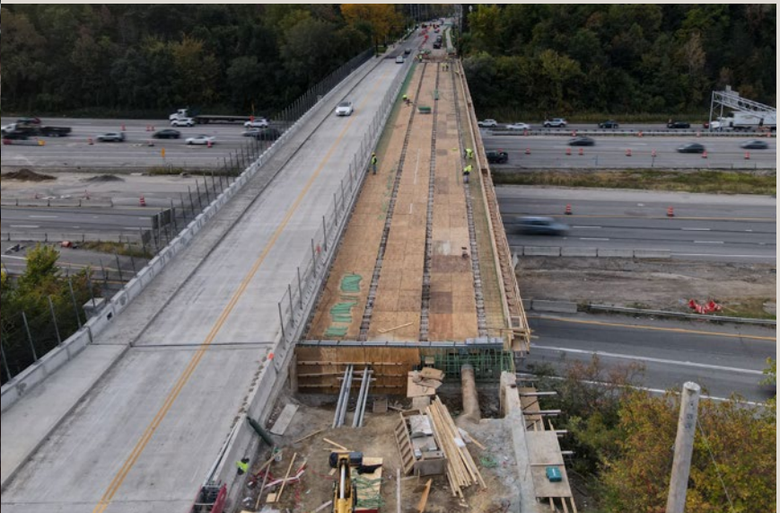
Aerial view of deck construction phasing
