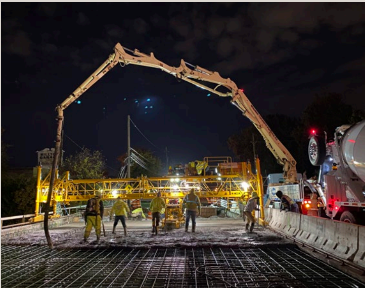
Overnight deck placement with phased construction
