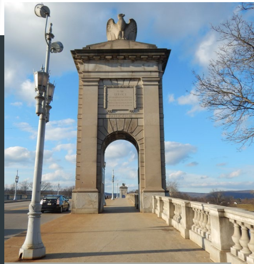
One of the four iconic pylons topped with an eagle carved from limestone Source: Greenman-Pedersen, Inc.
