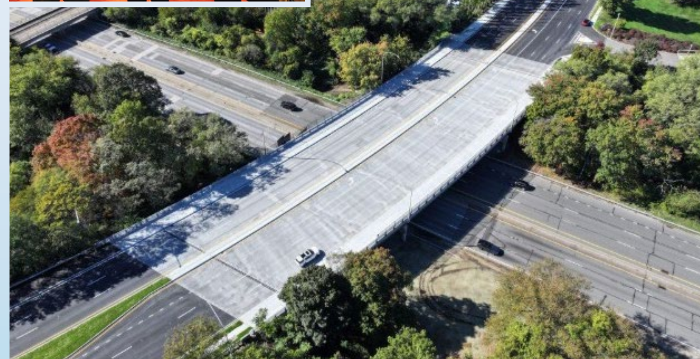
The rehabilitated Glenn Curtiss Boulevard Bridge
