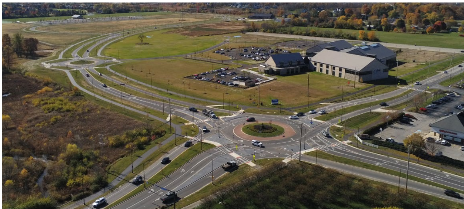
Aerial view of the completed roadway improvements demonstrating enhanced traffic flow, improved safety, and stronger pedestrian connectivity. Serving as a key gateway, the project supports a more walkable, connected community.
