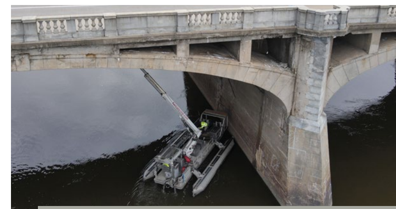
Top: Northeast side of the structure with one of two access points to Nesbitt Park and trails Bottom: In-depth, hands-on inspection work of Span 2, looking northeast Source: Greenman-Pedersen, Inc.
