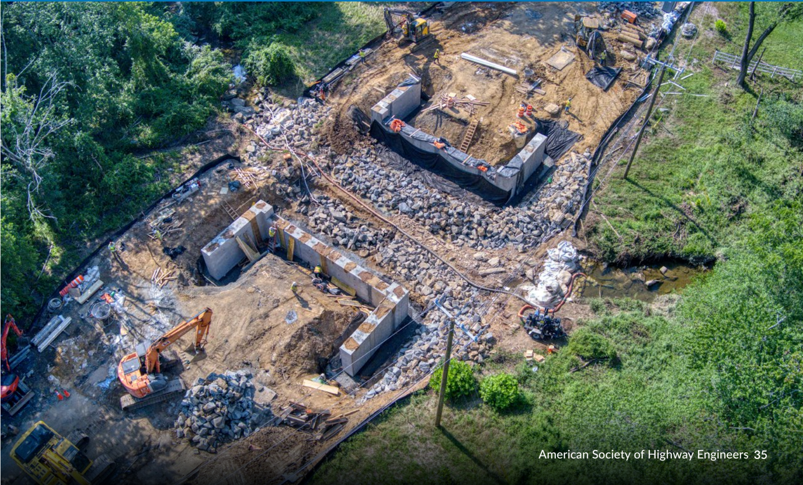
Aerial view of construction site after riprap placement
