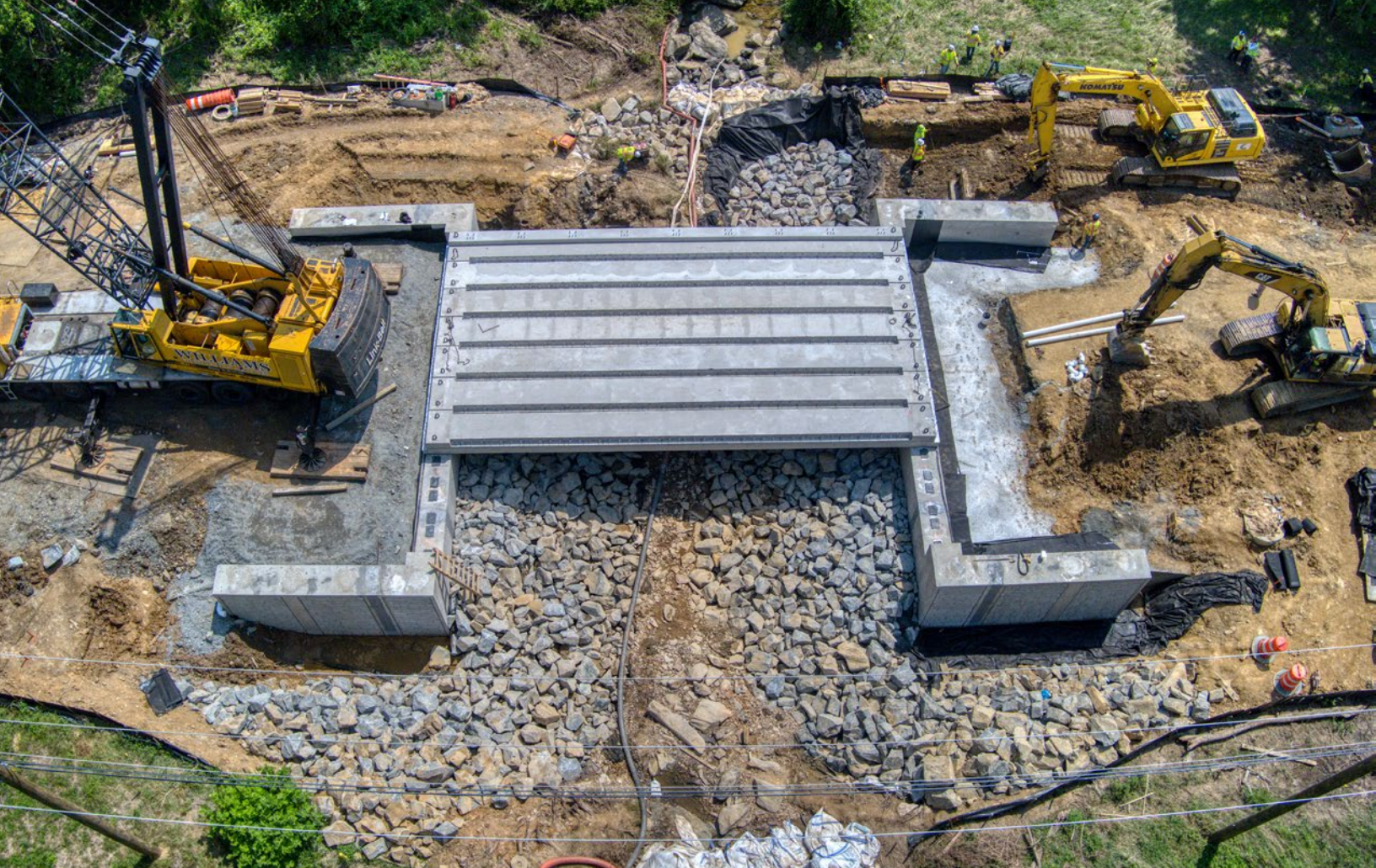
Top: Superstructure precast units being put in place Bottom: New bridge open to traffic during final construction stages
