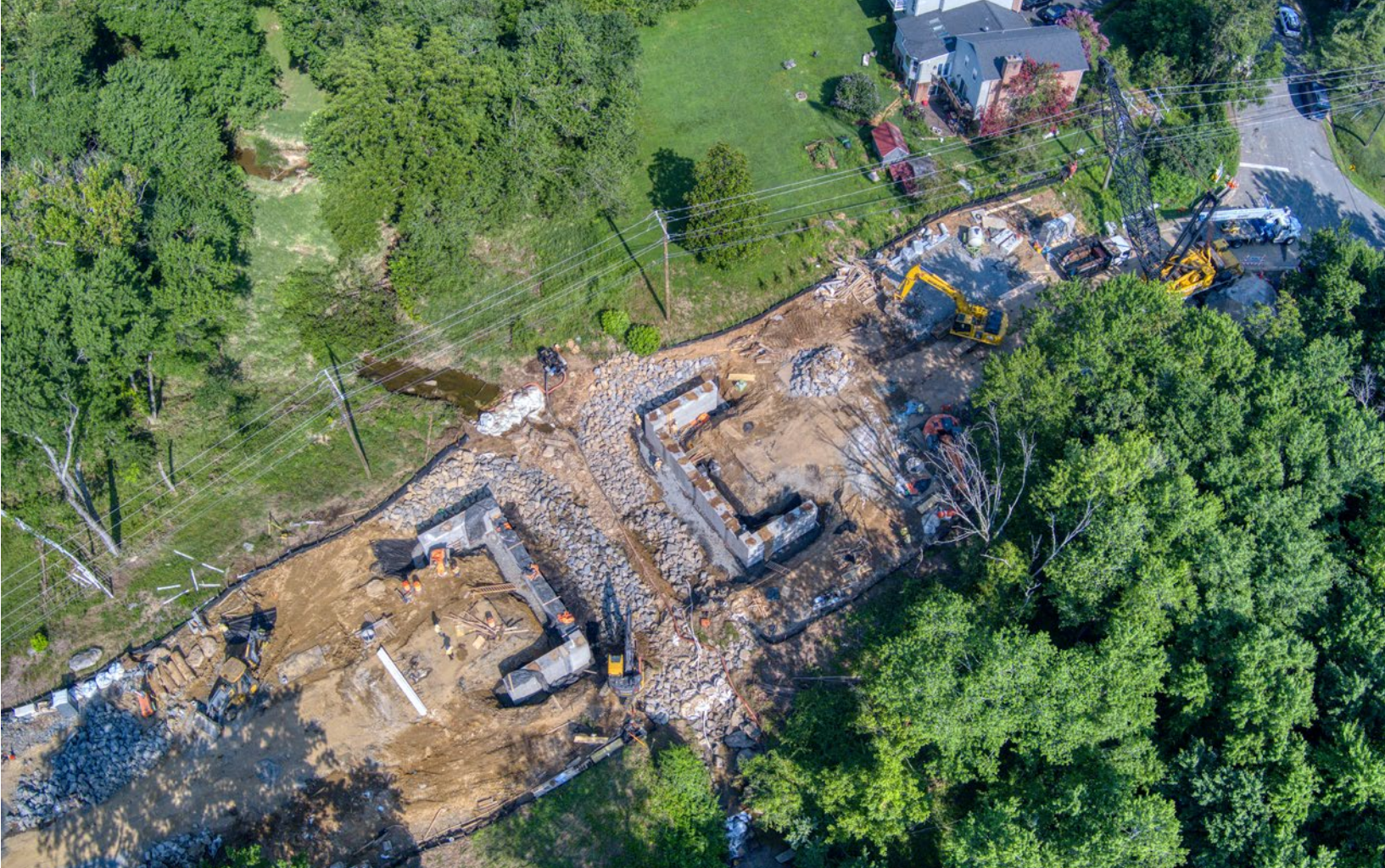
Aerial view of construction site after riprap placement
