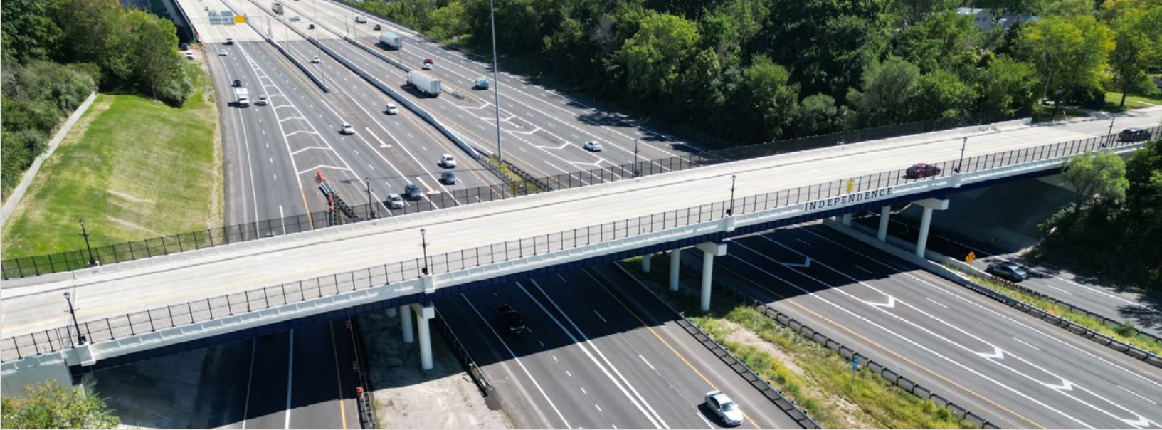
Finished Brecksville Road Bridge overlooking the completed I-480 Valley View Bridge
