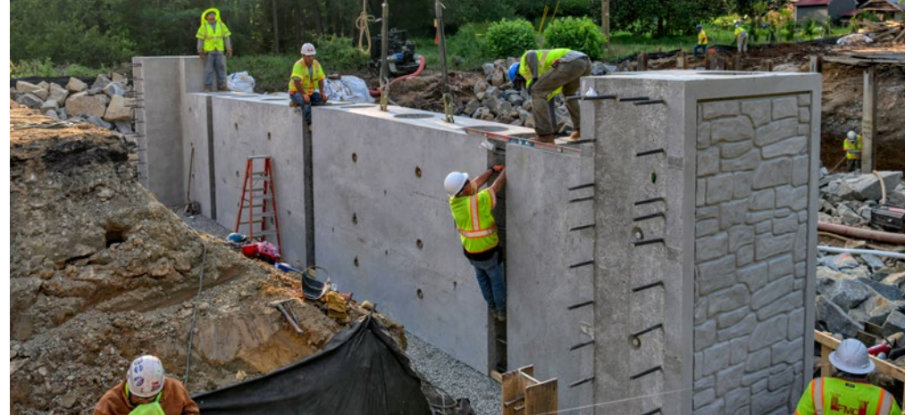
Installation of precast abutment units
