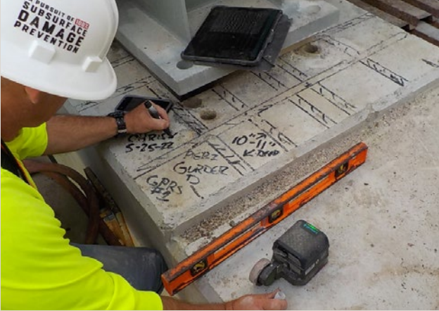
Locating pier cap reinforcement with GPR
