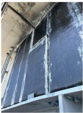
Carbon Fiber Reinforced Polymers strengthening the corbels
