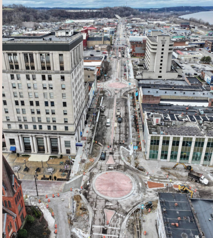
Construction of the mini-roundabouts at the intersections of 15th Street (background) and 16th Street (foreground)
