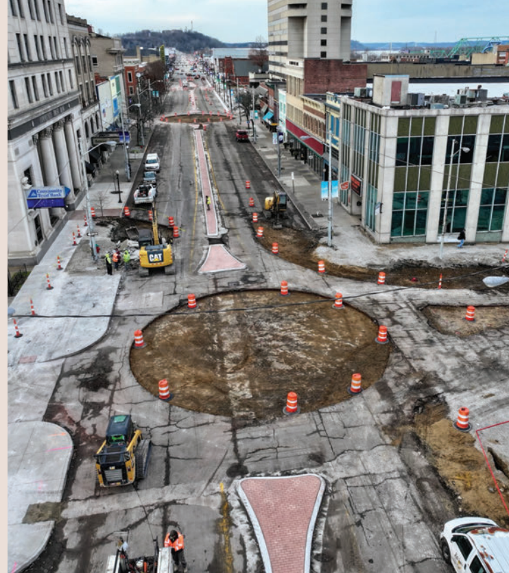
Construction of the mini-roundabout at the intersection of 16th Street
