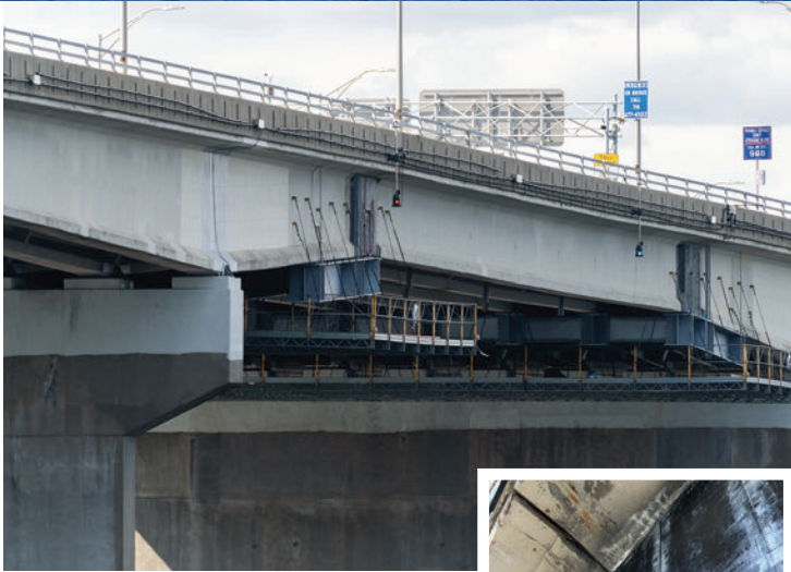
Redundant structural support system catches the bridge should the corbels fail
