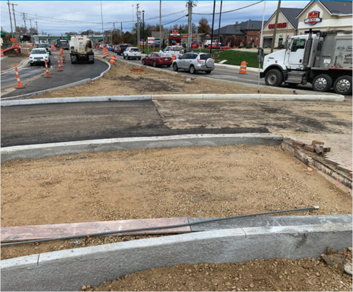
American Structurepoint engineers developed an intricate maintenance-of-traffic plan for the busy corridor that kept traffic moving while balancing safety for construction workers and motorists. Through carefully sequenced lane reductions, lane shifts and temporary pavement, the team maintained three open lanes throughout construction, minimizing disruptions for thousands of daily motorists. Credit: American Structurepoint staff
