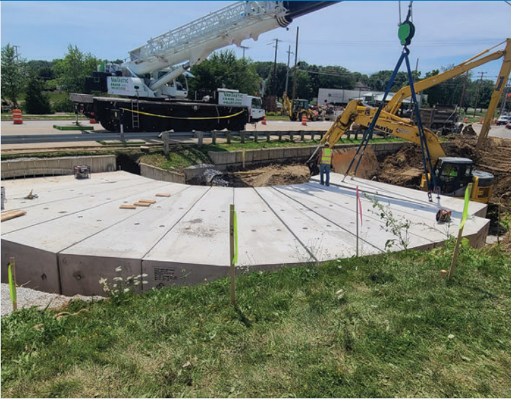
Installation of the uniquely S-shaped culvert at the Boettler Road and Massillon Road roundabout to convey a nearby stream underneath the new roadway. Credit: American Structurepoint staff
