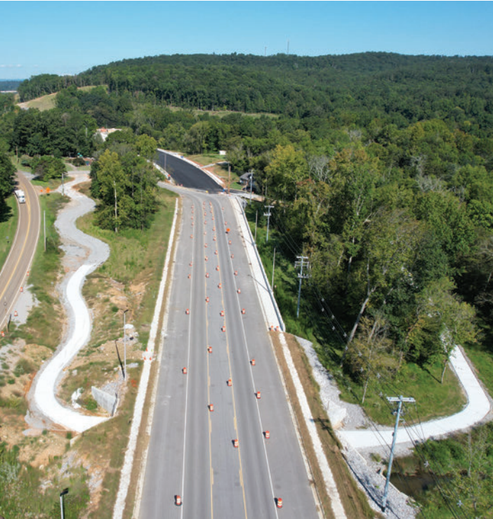
A tunnel was constructed under Apison Pike to provide a safe greenway connector removing the concern of pedestrians crossing the highway at-grade.
