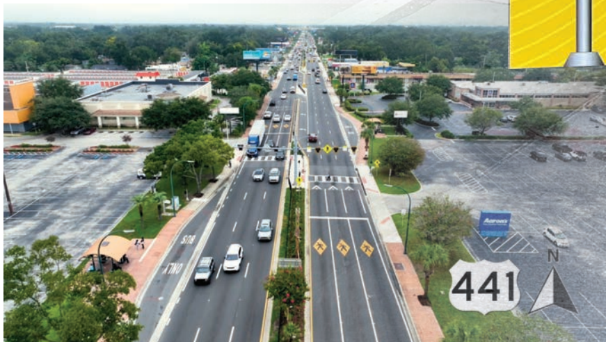
The Orange Blossom Trail (OBT) Pedestrian Safety Project in Central Florida is helping to save lives.
