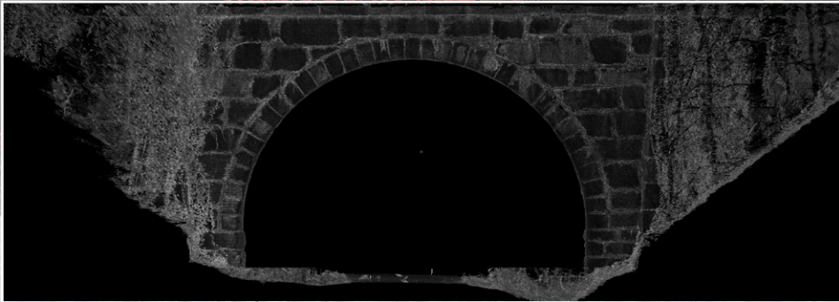
Project North-Western location as viewed using Leica Cyclone software
