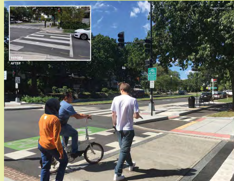
The design balanced the needs of the traveling public and those of the community, emphasizing pedestrian and bicycle safety.
