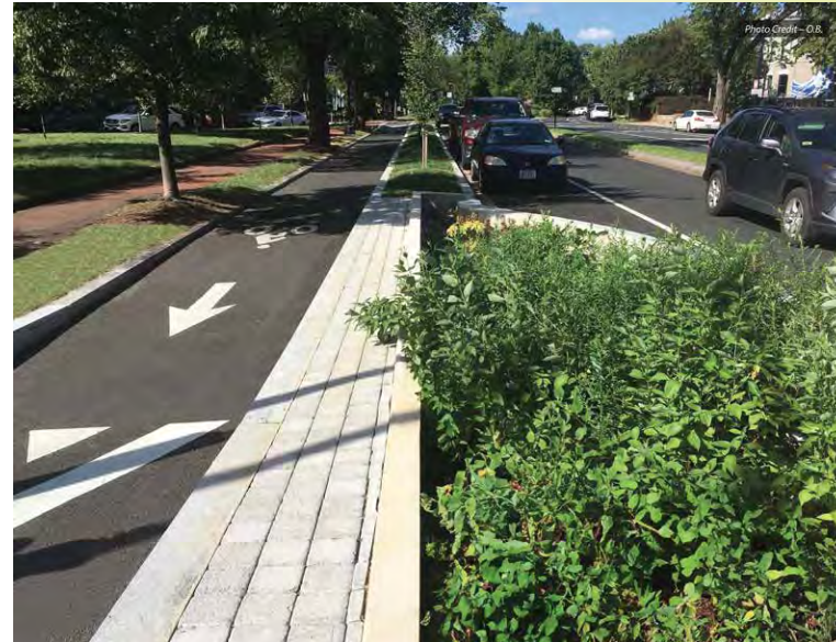
Curb extensions along the entire corridor help define parking and manage traffic.
