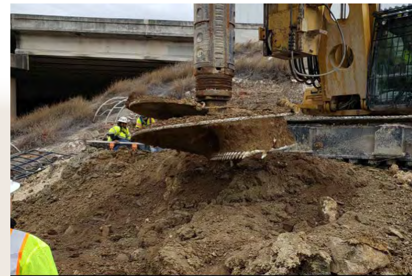
Figure 9: Bent 9 drill spoils at El. 668 to 670 (courtesy of Alamo NEX Construction)
