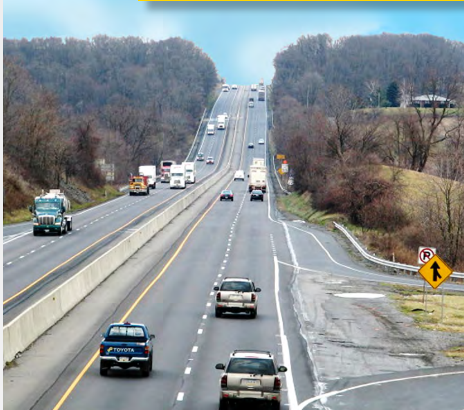
Roadway prior to improvements
