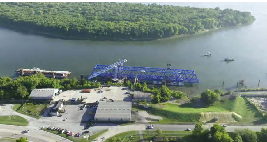
Truss span at the Paducah Riverport Facility on the morning of the float
