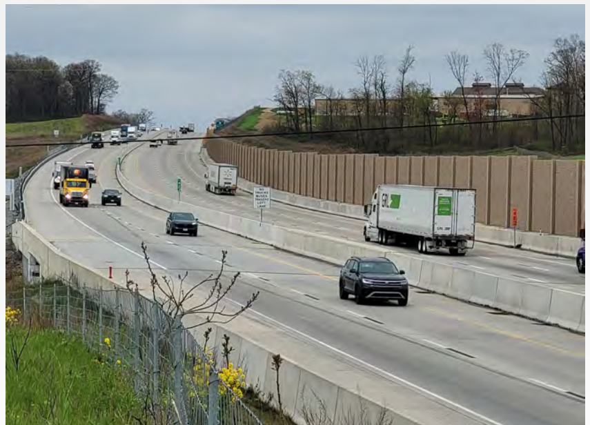
Westbound truck climbing lane
