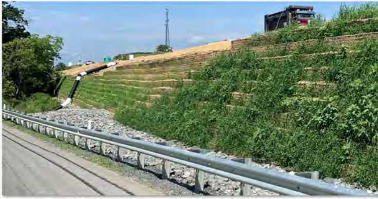
Geosynthetic reinforced slope
