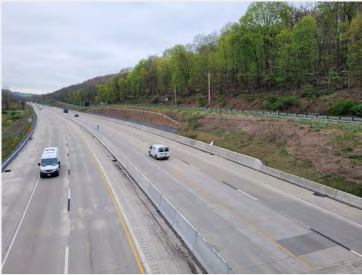
Completed roadway section
