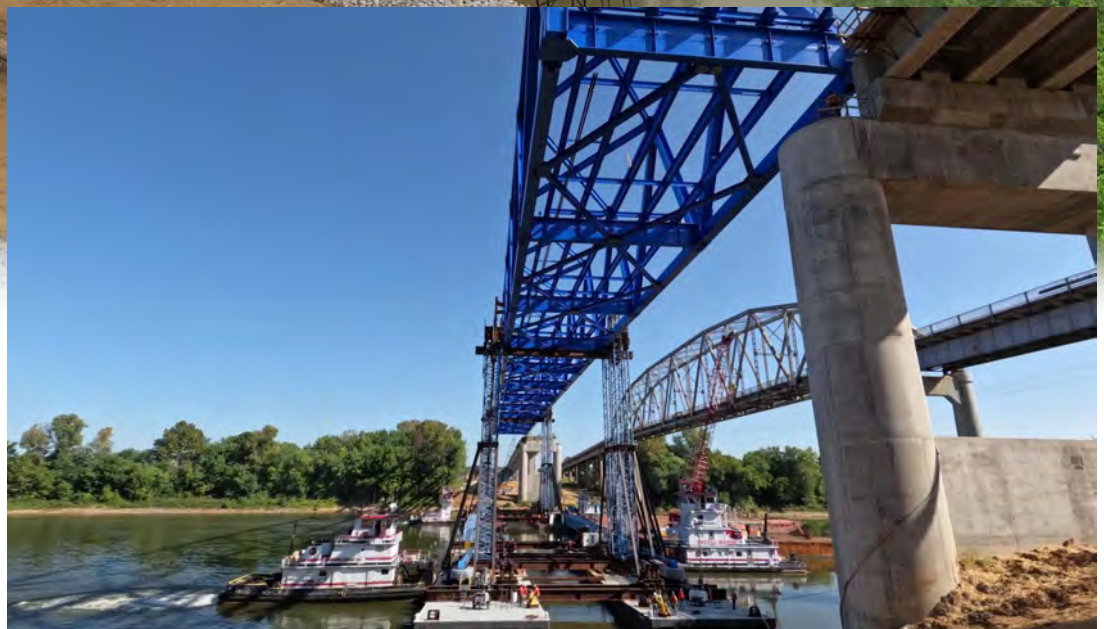
Truss span moving into place after reaching lifting height
