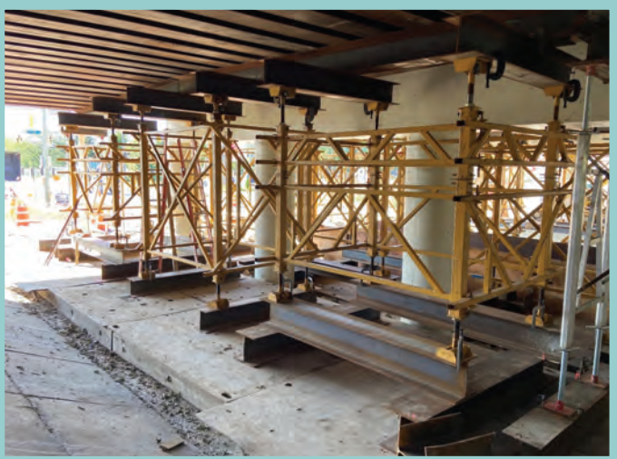
Phase Four temporary shoring for the concrete bridge slab
