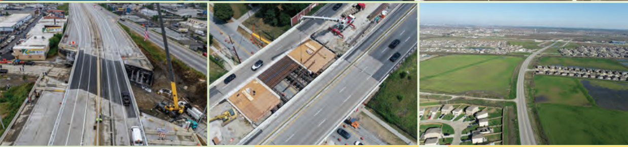
6 Emergency Repairs to I-95 Bridge
