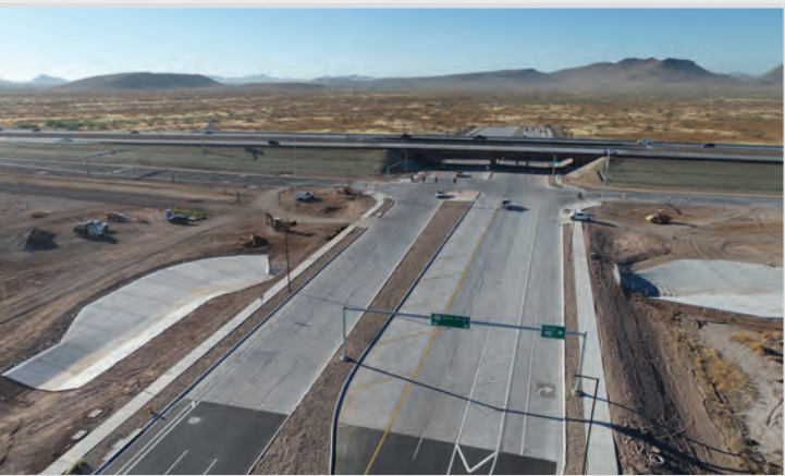
Completed Loop 303 traffic interchange at 43rd Avenue
