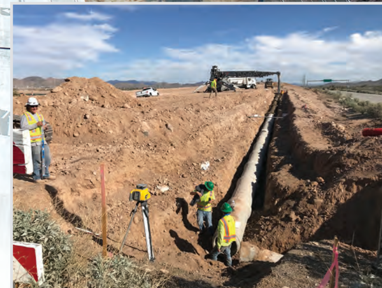
Application of slurry backfill at all storm drain pipes, bridge footings and abutments saved labor costs compared to manual placement of aggregate.
