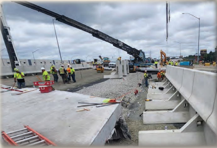
Placing Gravix barriers
