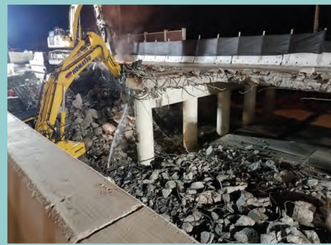
Concrete bridge slab demolition with Worden Road closed underneath
