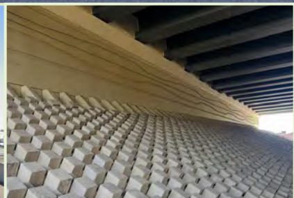
38 Rebuilding I-95 Section BS1 Interchange
