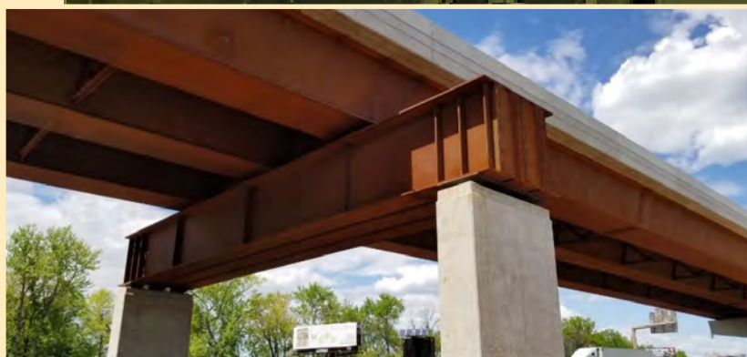
Ultra-high performance concrete closure pour
