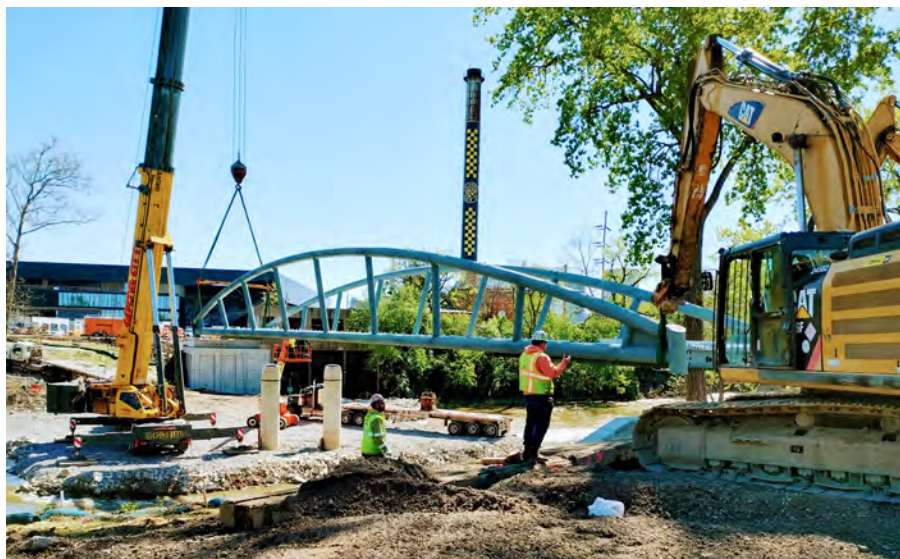
Each span was lifted into place fully assembled during construction.
