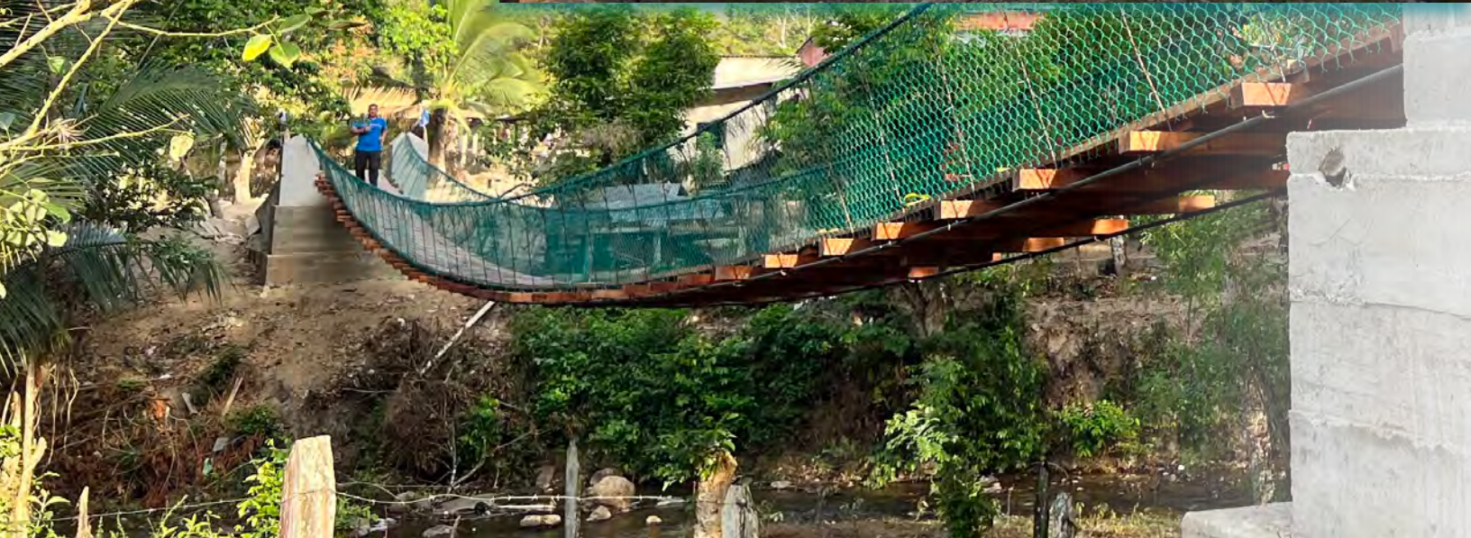
The Peugeot Center volunteer team, Predisan employees and community members celebrated the bridge's opening in 2023.
