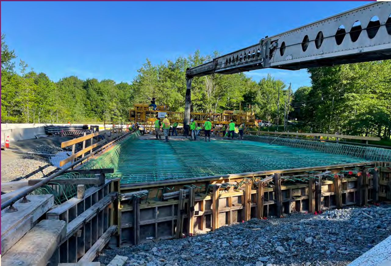
June 2021, bridge deck concrete pour
