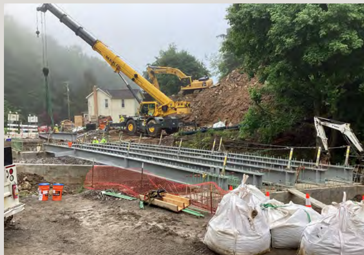
A crane near two residences assisted with beam placement for the new bridge.
