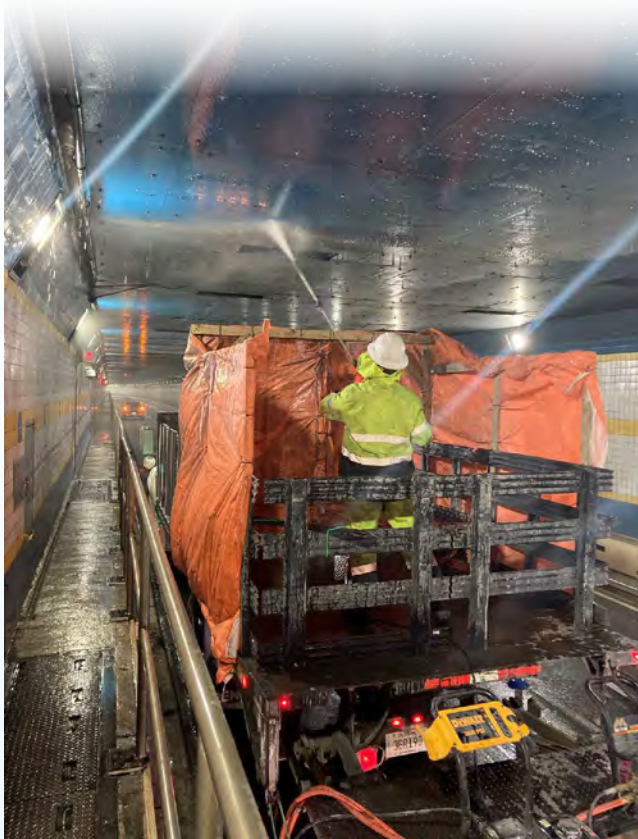
Tile cleaning of the Queens Midtown Tunnel
