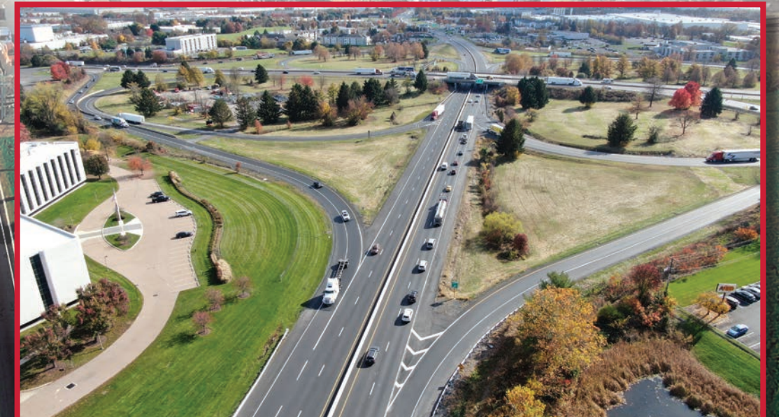
Completed SR 100 and I-78 interchange, looking south
