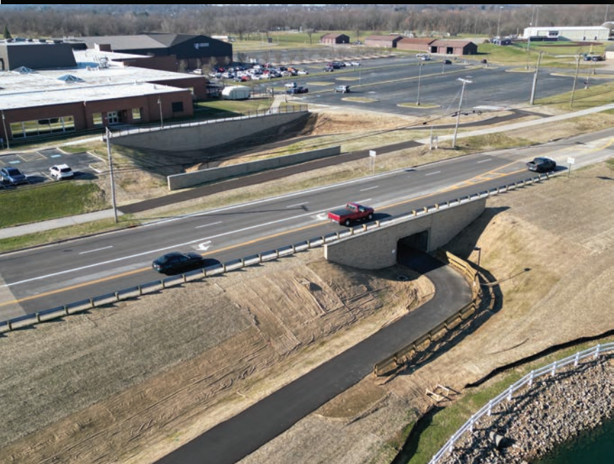
Finished construction, looking southwest
