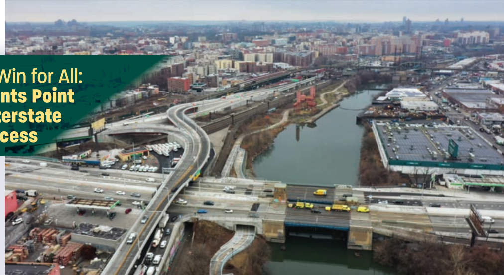
New Bruckner Expressway dual viaduct entrance/exit ramp to and from Edgewater Avenue and Hunts Point Peninsula. The view, looking north, shows connection to new Sheridan Expressway and Concrete Plant Park along Bronx River.
