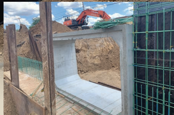
North headwall at start of construction
