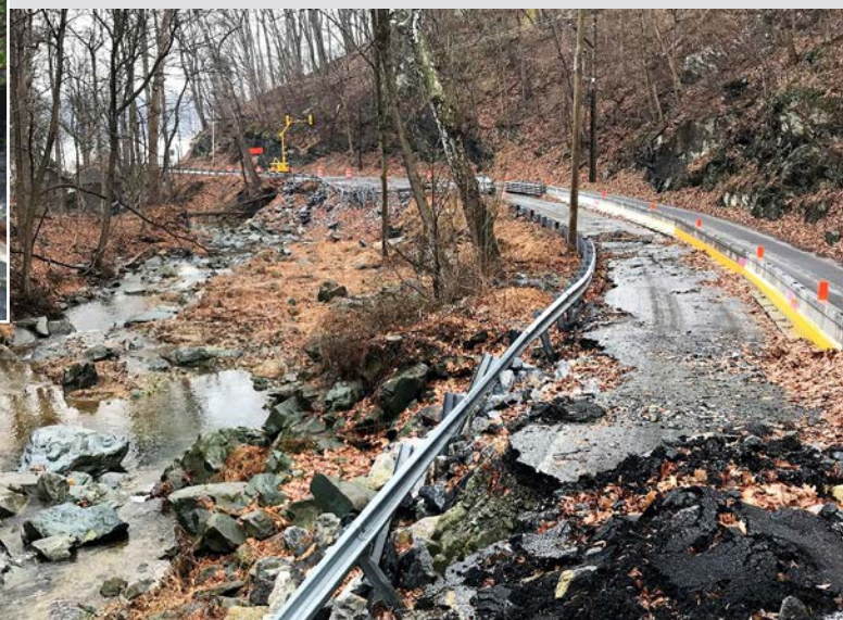
Eastbound view of roadway during single lane traffic operations; lane protected with temporary signal system (background) and temporary barrier system
