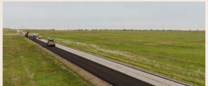
CIP pavement placed and compacted on ND 8 Courtesy of Midstate Reclamation, Inc.
