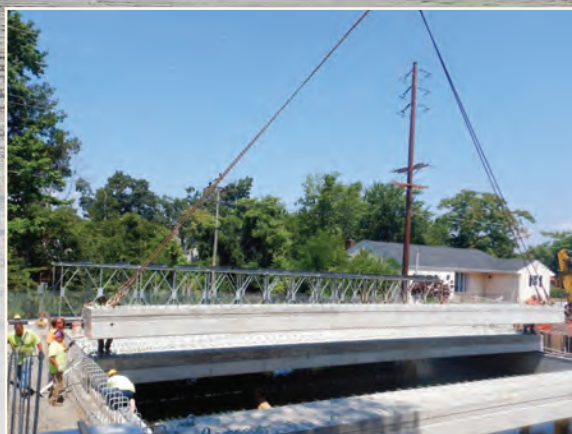
Box beam placement construction with Acrow bridge to provide access for pedestrians
