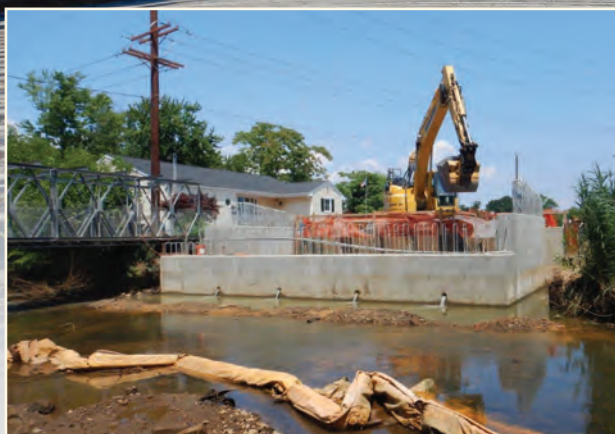
North abutment under construction with Acrow bridge to provide pedestrian access
