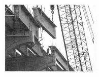
beams was post-tensioned. This post-tensioned section is 900' in length and 175' above the floor of the Cuyahoga Valley.
