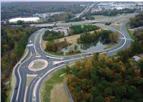
I-95/Temple Avenue Interchange Under $20M Winner Owner: Virginia Department of Transportation Engineer: Rinker Design Associates, PC Contractor: EV Williams
